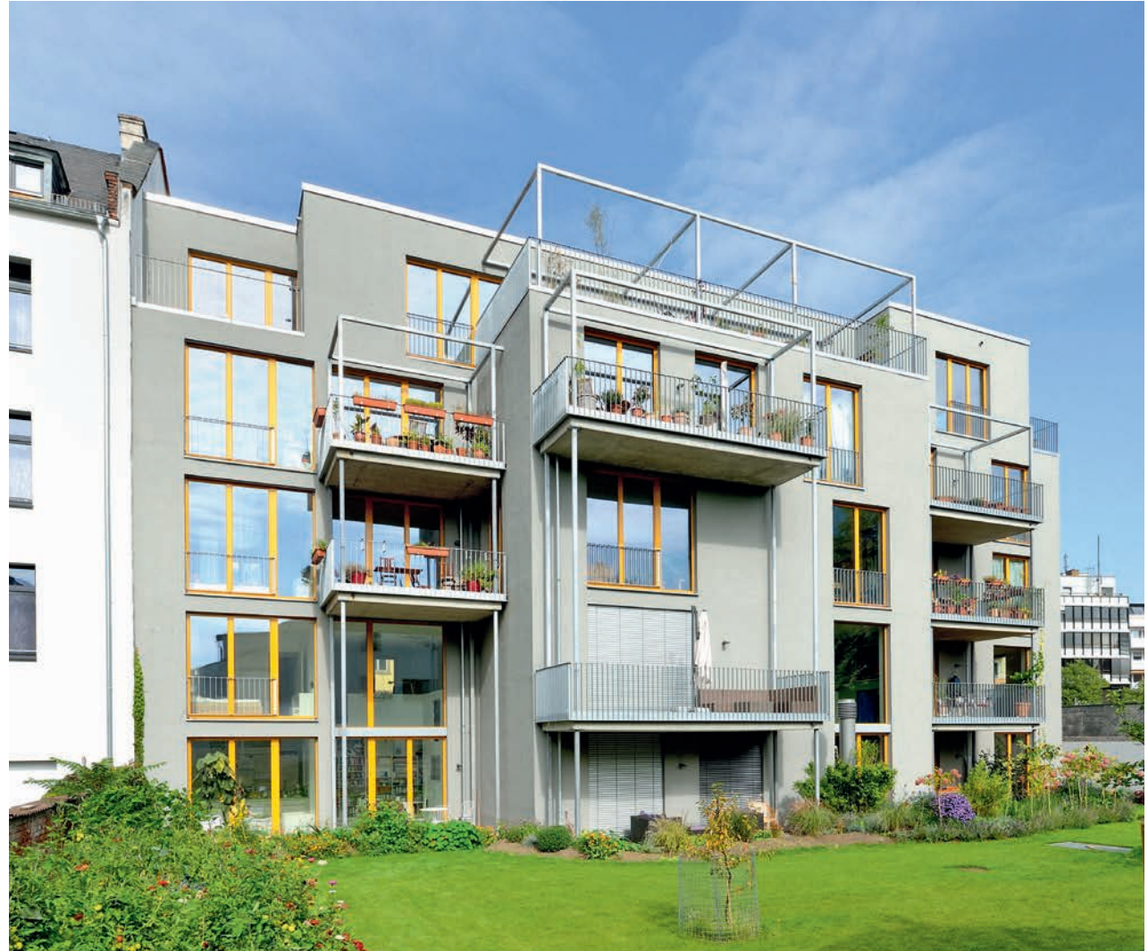
bouwgroep Ostend Residential Building, Frankfurt
